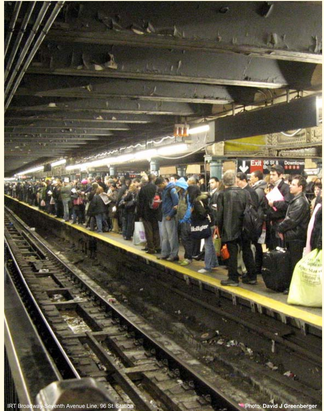
IRT Broadway-Seventh Avenue Line, 96 St. Station
