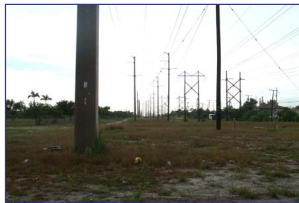
Florida Power & Light Right of Way Looking West from SR 710
