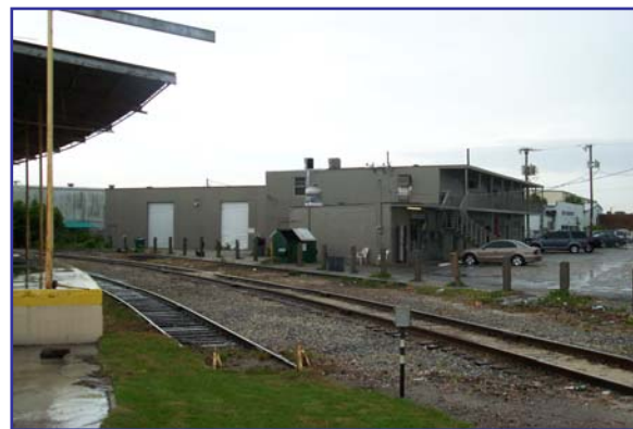
Lewis Terminals Track and Commercial Buildings along SR 710, Looking North
