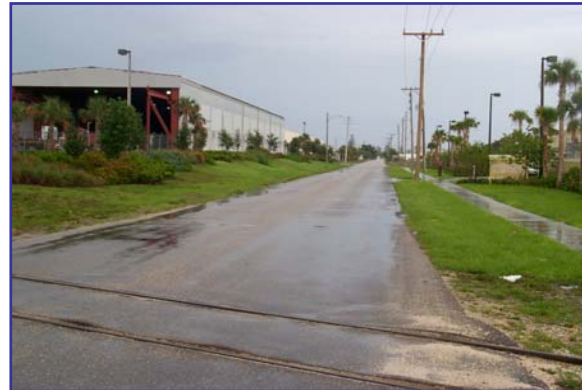
Looking East on West 13th Street From Existing At-Grade Crossing
