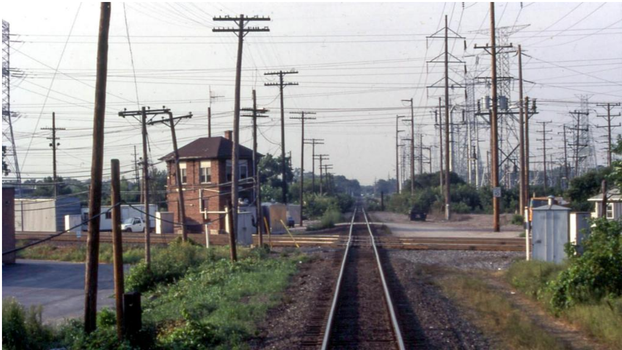
9 10 11 Figure 18. Deval Crossing, seen from a North Central Service train just north of the CNW Northwest Line, 1990, 12 David Wilson photo (CC BY 2.0). 13 14
